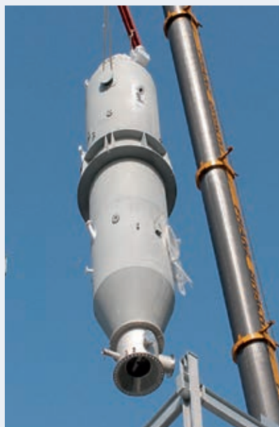
Assembly of a complete, pre-lined combustion chamber with attached, flanged air/water quenching head
